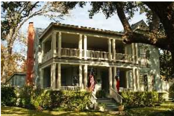
The old Coronal Institute's one room classroom has been expanded through the years by its different owners to accommodate their families to its current two-story size for Donna and Gerald Hill. Photo by Linda Kees
