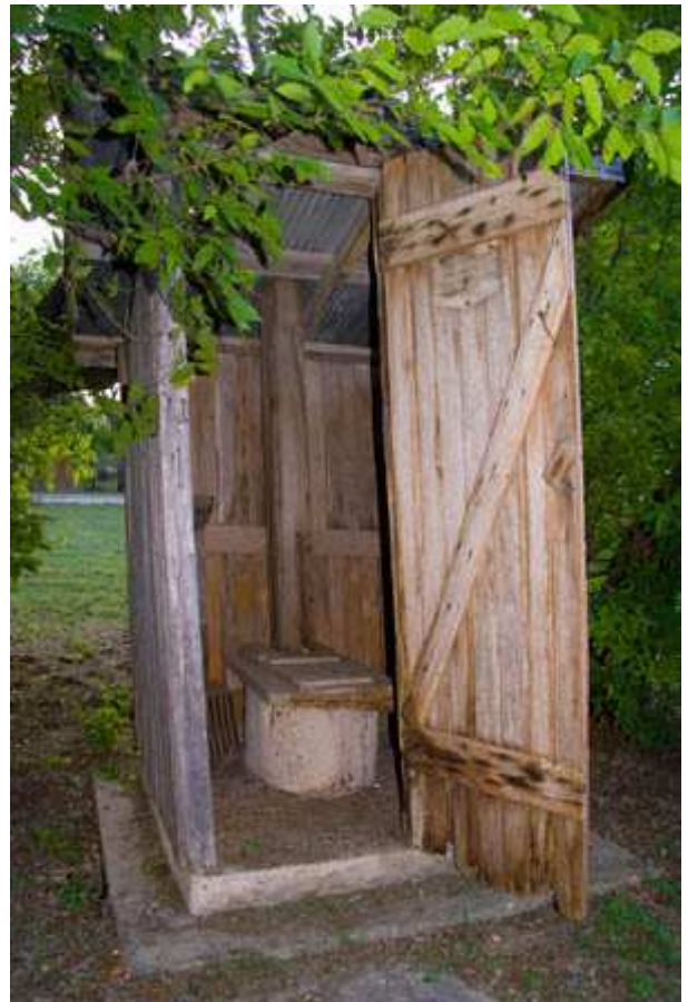
Driftwood general store outhouse built by W.P.A. in 1938.
